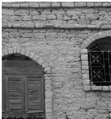
Masonry cornice lines
