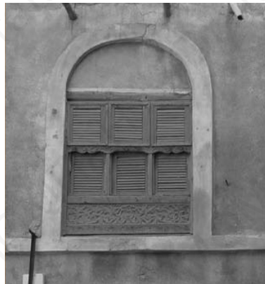
Blocked in arched window
