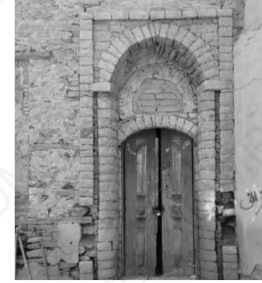
Arched masonry entrance
