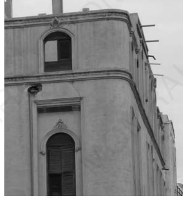
Timber fence parapet
